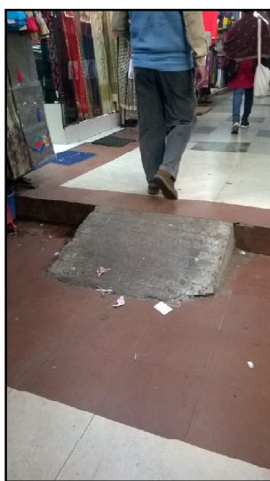
Picture 5: Ramps and Access: New Market
